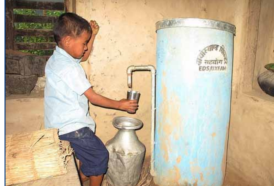
7 yr old Shanta Rame Ale using a water filter recently installed in the family home Image: Oxfam International
